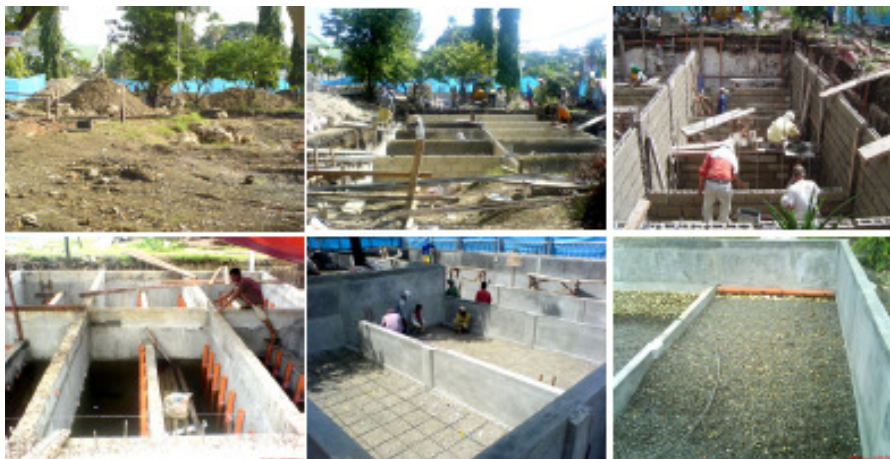
Figure 4: DEWATS Construction
