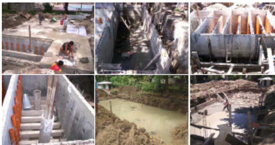
Figure 5: Construction of the DEWATS. (Source: BORDA)
