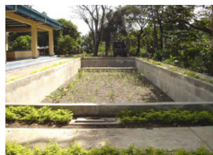
Figure 2: View of the aerobic treatment modules: planted gravel filter (PGF), indicator / polishing pond (IP). (Source: BORDA)
