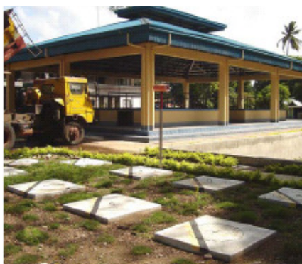
Figure 1: View of the anaerobic treatment modules: settling tank (ST), anaerobic baffled reactor (ABR) and anaerobic filter (AF). (Source: BORDA)
